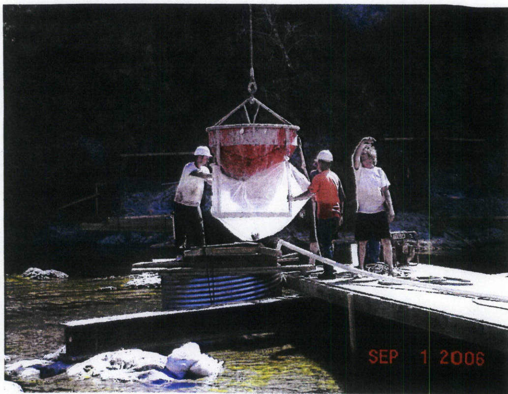
Figure 4c. Setting cement seal pour in culvert pipe coffer. Note plastic sheet at bottom to minimize cement introduction to mainstem .
