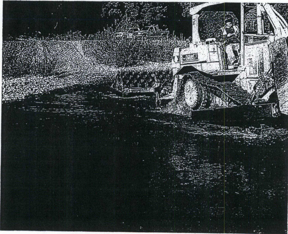
Figure 40. Wet-channel crossing number 2. Bulldozer with sheep-foot roller attached.
